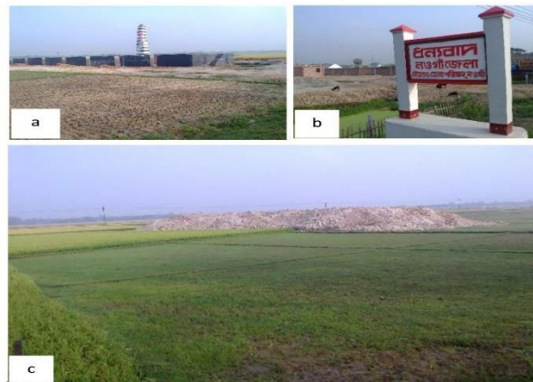
Fig. 6: Photograph Showing (A, C) Land Degradation Due to Construction of Brick Field in the Irrigated Area, (B) Land Degradation by Cutting and Filling of Soil for the Construction of Industry and Housing.
