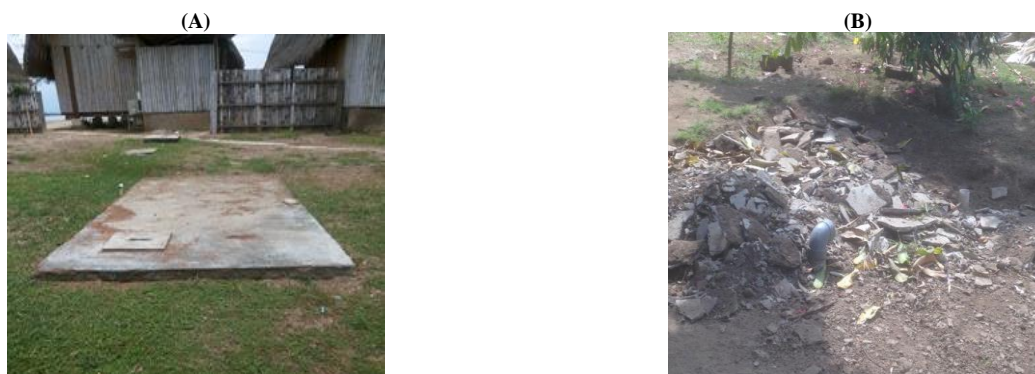
Fig. 2: An Example of A Septic Tank. Remarks: A. Septic Tank in the Hotel Area; B. Septic Tanks in Residential Areas.
