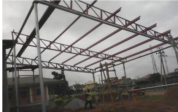
Plate 2: Installation of Trusses and Z Purlins.
