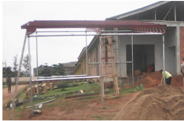
Plate 1: Erection of Poles.
