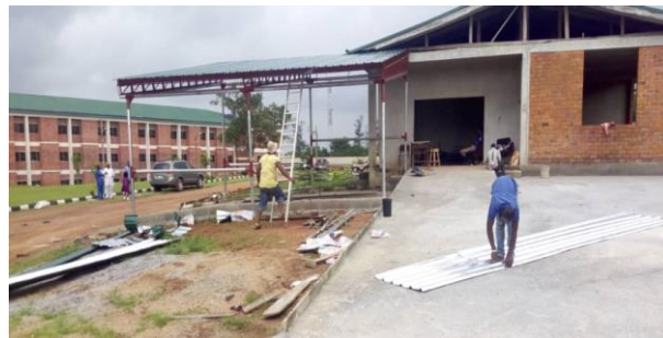
Plate 3: Roofing in Progress.
