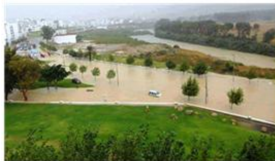
Fig. 10: Urban Damages Caused by Heavy Rainfall during the Morning of the August 29, 2013 in City Of Tetouan
