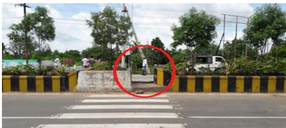
Fig.18: at chainage: 268.817km.
