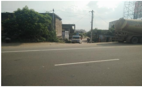
Fig.24: at chainage: 254.017km RCW.
