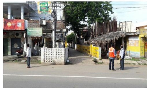
Fig.23: at chainage: 269.260km. RCW
