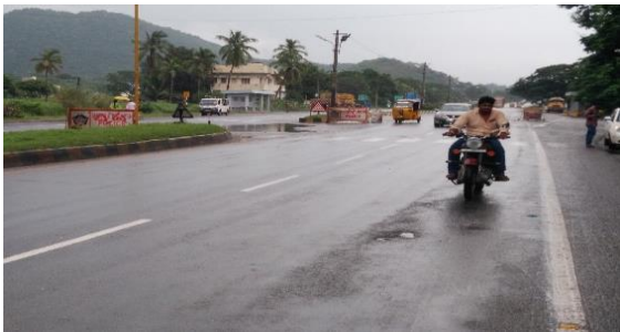
Fig.17: at chainage:256.125km RCW.
