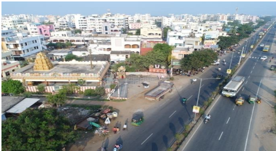
Fig.25: at chainage: 267.193km.
