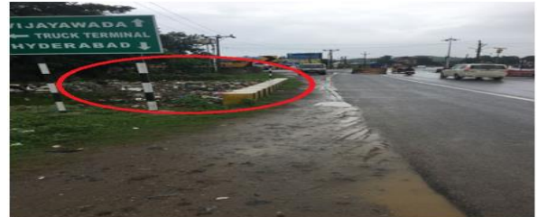
Fig.9: at chainage: 256.720km LCW.
