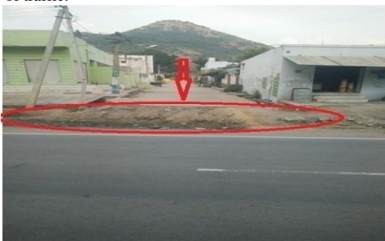
Fig.27: at chainage: 247.915km.LCW
