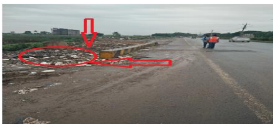
Fig.7: at chainage: 258.220km RCW.
