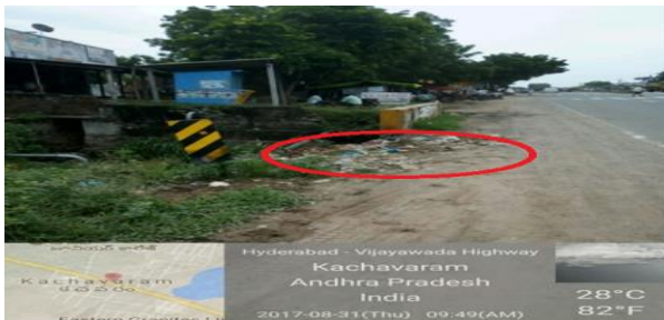
Fig.10: at chainage: 249.756km LCW.
