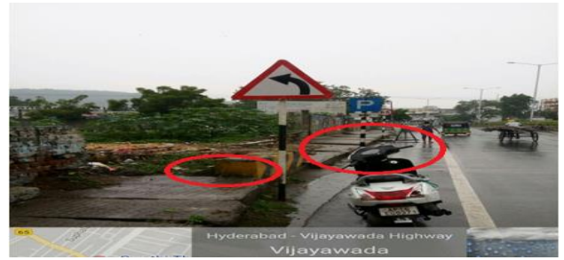
Fig.19: at chainage:269.557km. LCW
