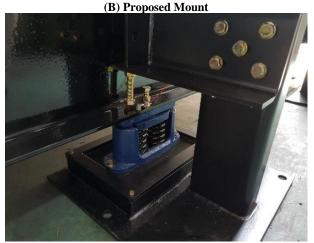
Fig. 2: Passive-Type Mount Module for Electric Power Plant.
