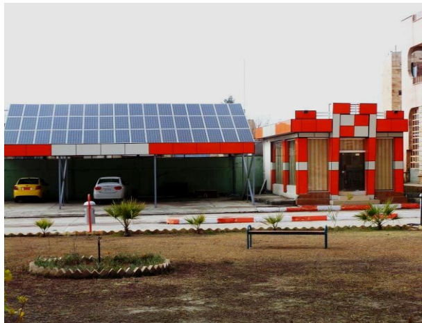
Fig. 12: Technical Collage of Mosul / Solar Power Plant.
