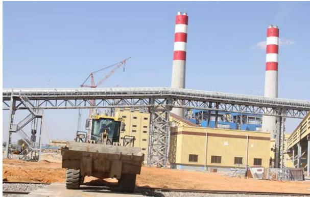
Fig. 4: Morulae A Power Station- Under Refurbishment.
