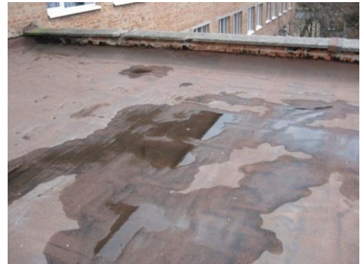
Fig. 1. The main typical defects of combined roofs: a, b) brickwork destruction of walls in places of external drainage; c) destruction of the parapet brickwork; d) destruction of parapet plates; e) separation of the coating carpet; f) leakage of the carpet covering in places of metal racks installation, outlets of sewer risers, etc.; g) destruction of bitumen coating on roof superstructures; h) violation of the drainage gradient and the formation of drainage areas.
