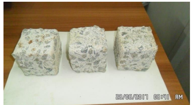
Fig. 2. Concrete cubes deteriorated due to H 2 SO 4
