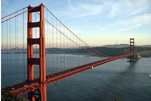
Fig.4. Golden Gate Bridge
