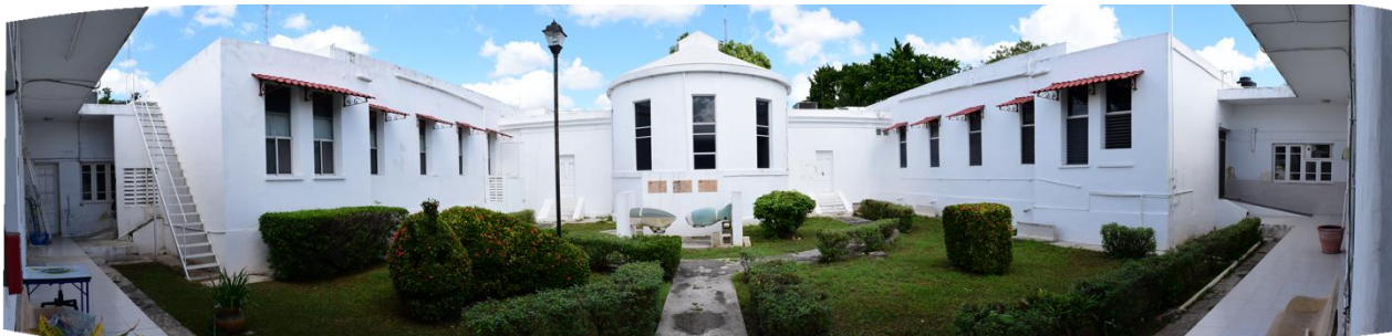
Fig. 6: View to the interior garden.
