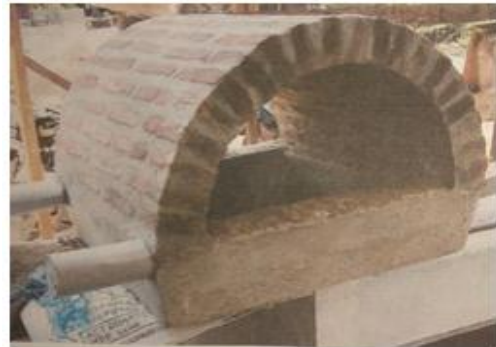
Fig. 7: Vault after removal of formwork
