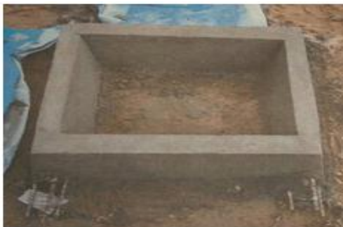
Fig. 3: Base after Concreting
