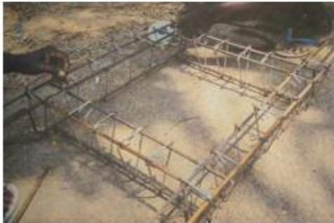
Fig. 2: Reinforcement for base
