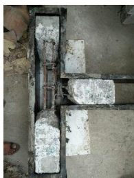
Figure 5: Specimen after chipping
