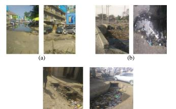
(c) **Figure 8**a: poor drainage in Ibrahim Taiwo road; 8b: open and clogged drainage in Abattoir area and; 8c: blocked and poor system of drainage along IBB road (source: fieldwork).
