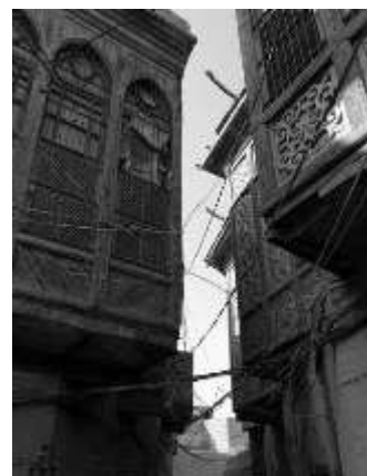
Figure 3: Physical observation, wooden lattice windows ( Shanashheel ), adjacent context Source: Author
