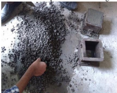
Fig 3: Mixing of concrete
