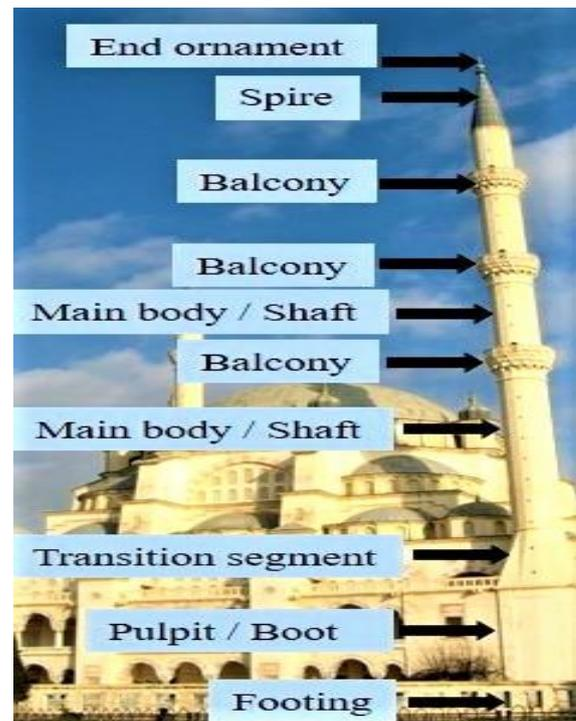
Fig. 1: Component Segments of an Ottoman Minaret.
