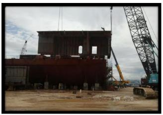
Figure 6: Picture of Module (Lifting Process) [10].
