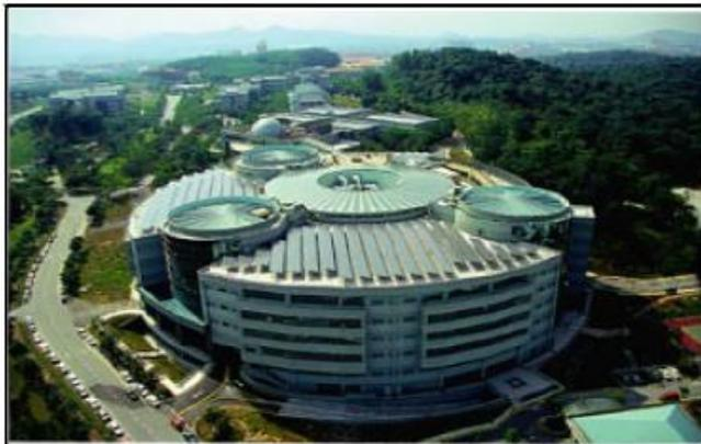
Fig 2: The largest of GCPV System with 361.9 kWp at Enterprise Four Building, Technology Park Malaysia (TPM), Malaysia (Source: TPM)
