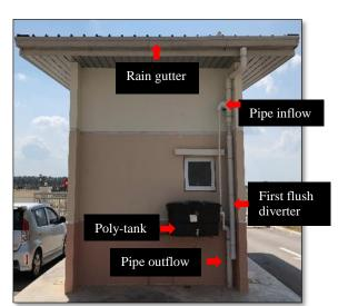
Fig. 3: Complete installation of Smart Kit RWH system
