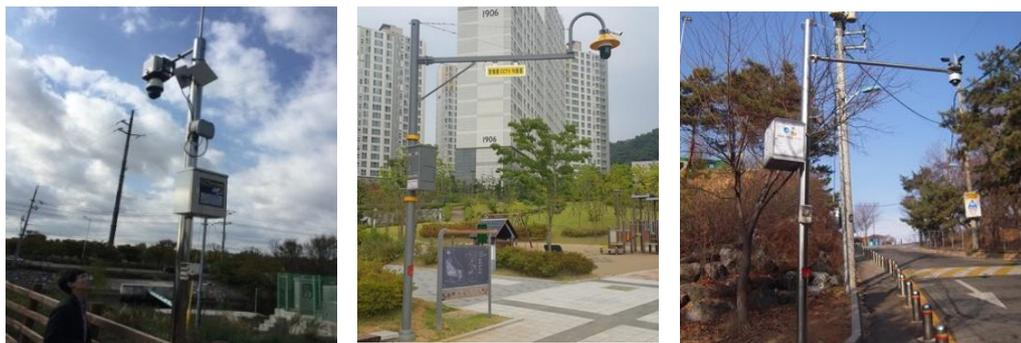
Figure 2: Control units installed to poles with CCTV cameras
