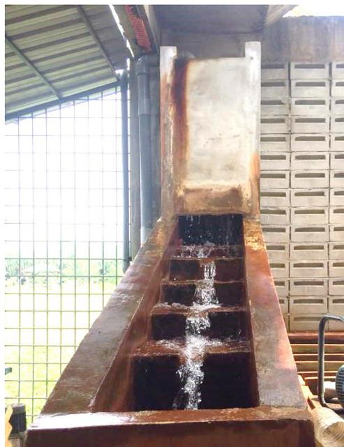
Fig. 2: Concrete stepped cascade aeration
