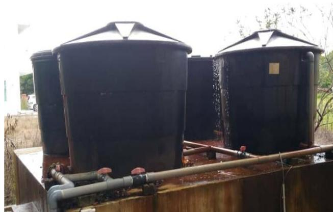
**Fig. 5:** HDPE tank for treated groundwater
