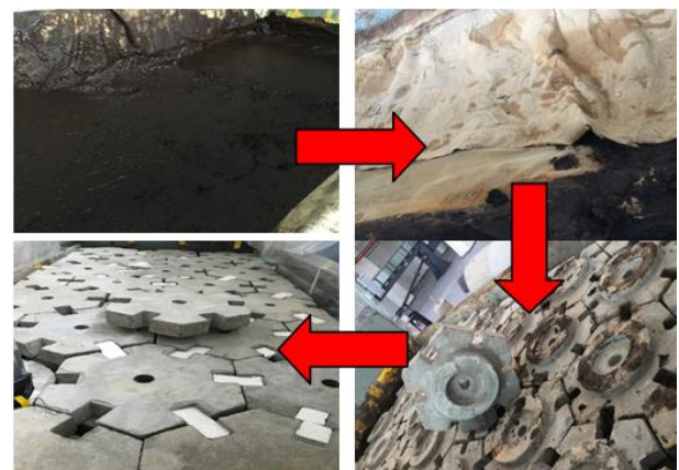
Fig. 2: Installation Process of CDP on the Peat Soil.
