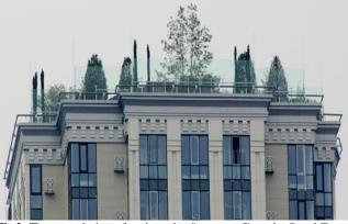
Fig.2: The general view of an intensive "green roof" on the *Royal Tower* residential complex (Kiev)
