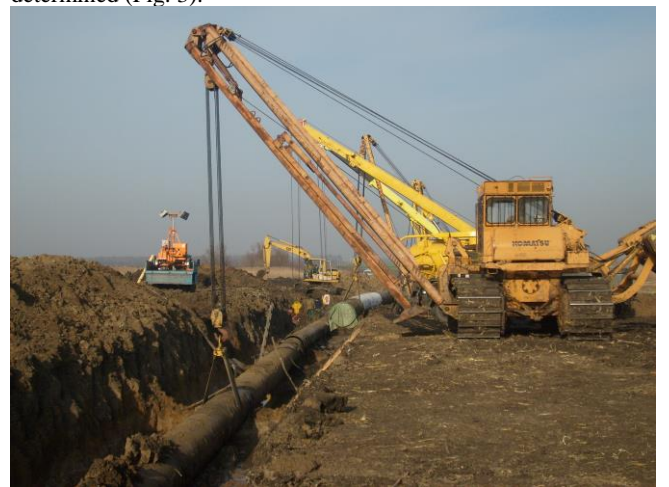
Fig. 2: Main oil pipeline new section installation
