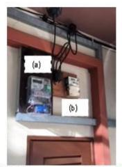
Fig. 3: (a) PV export meter and (b) TNB meter.
