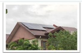
Fig. 1: Photovoltaic modules mounted on rooftops (Retrofitted GCPV System).
