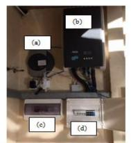
Fig. 2: (a) The inverter, (b) solar log data logger, (c) AC junction box and (d) DC junction box.
