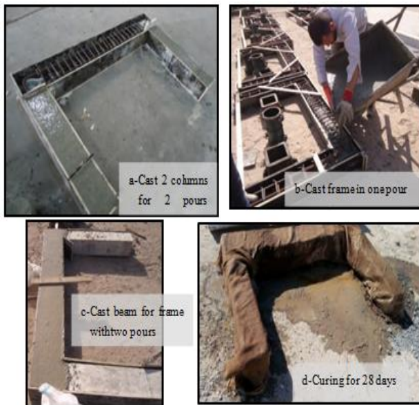
Fig. 5: Concrete casting and curing steps
