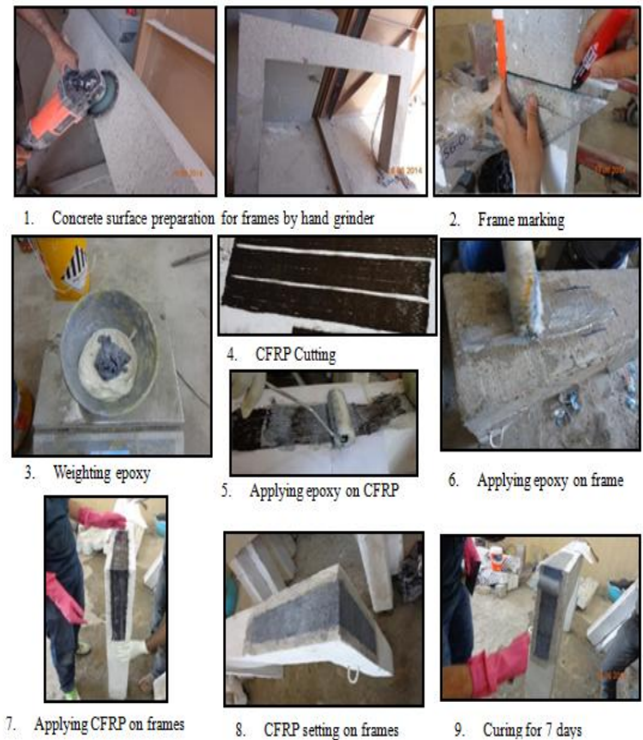
Fig. 6: CFRP- sheet setting on frame
