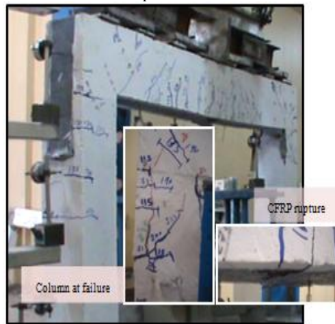
Fig. 10: Crack pattern for frame Fu-S
