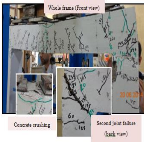
Fig. 12: Cracks pattern for frame (Fu-2P)
