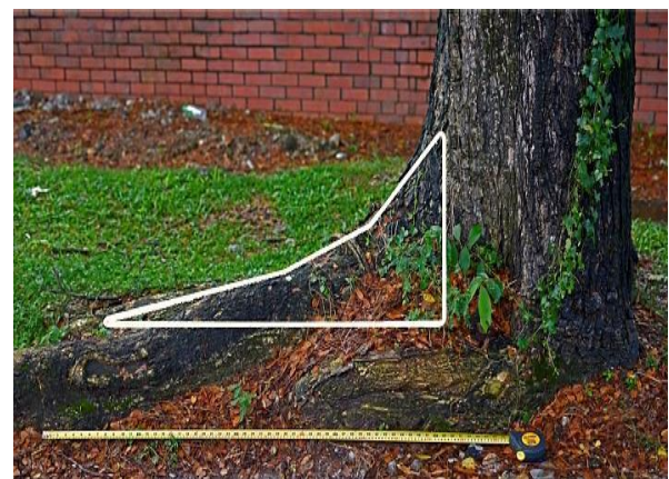
Fig. 1: The shape profile of Method of Tensile Triangles follows closely to the shape of buttresses.
