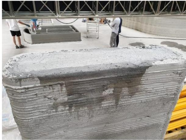
**Fig. 14:** Concrete casted within 5cm 3D printed walls.
