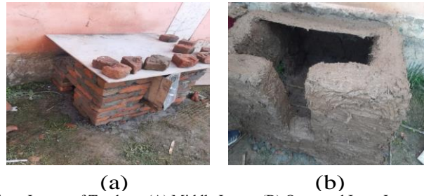
Fig. 6: Three Layers of Tandoor: (A) Middle Layer, (B) Outer and Inner Layer of Tandoor.
