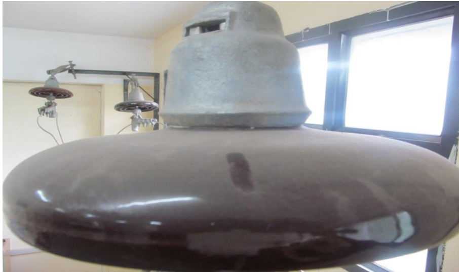
Fig. 9: Above Fig Indicate the Set Up at Location -1.
